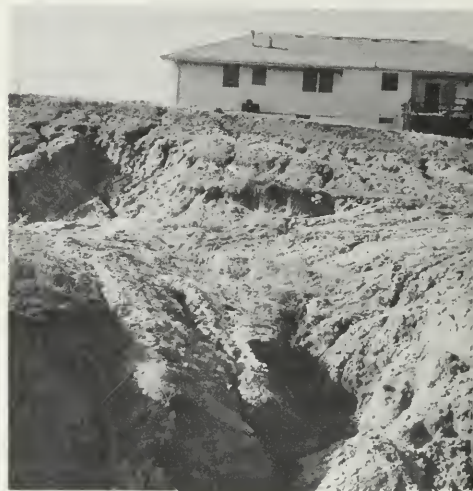
Developer of apartment complex above in Indianapolis used an excavated area for storm water storage, recreation, and for scenic value. Storm water is routed into this area and released through an outlet at a retarded rate. Right, improper disposal of surface water caused gully threatening a home in Des Moines. Below, sediment and debris fill channel of small stream where it passes through a development in Washington State.
